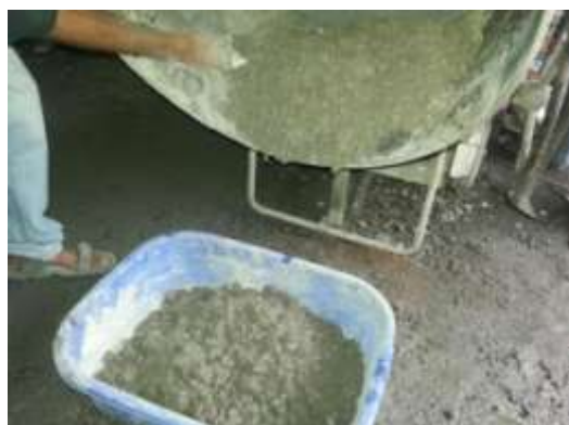
Fig.1 Mixing of Constituent materials
